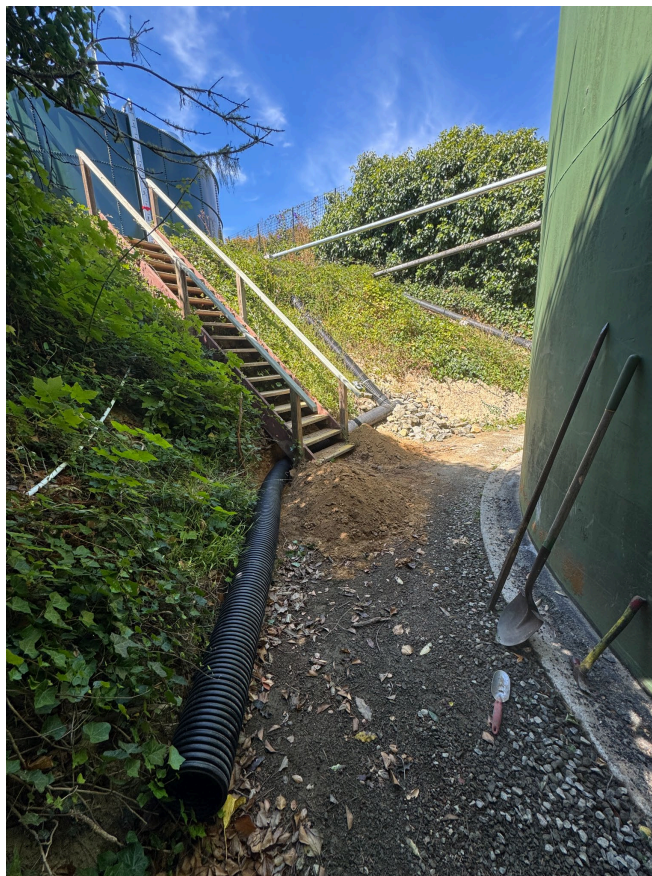
Photo 2. Completed drainage routing along tank access area, with corrugated pipe installed along the tank/stair corridor.
