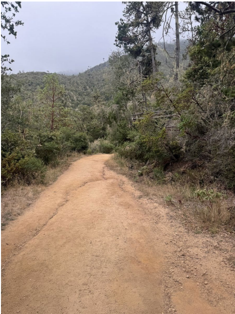
Photo 9: Erosion, failed drain, debris, and overgrowth
