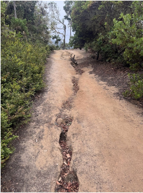
Photo 7: Erosion from failed drains and water bars
