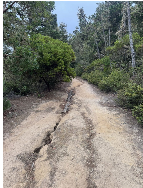
Photo 10: Extensive erosion from failed systems
