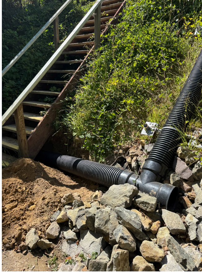
Photo 3. Completed drainage piping and tie-in area adjacent to the tank access stairs, with rock and soil restoration visible.
