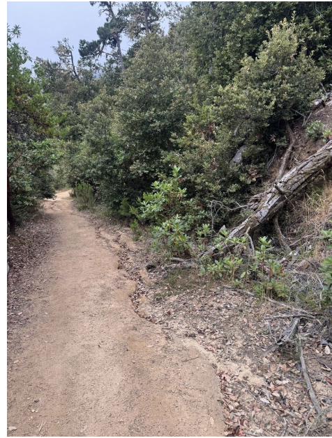
Photo 8: Failed in-slope drain and overgrowth
